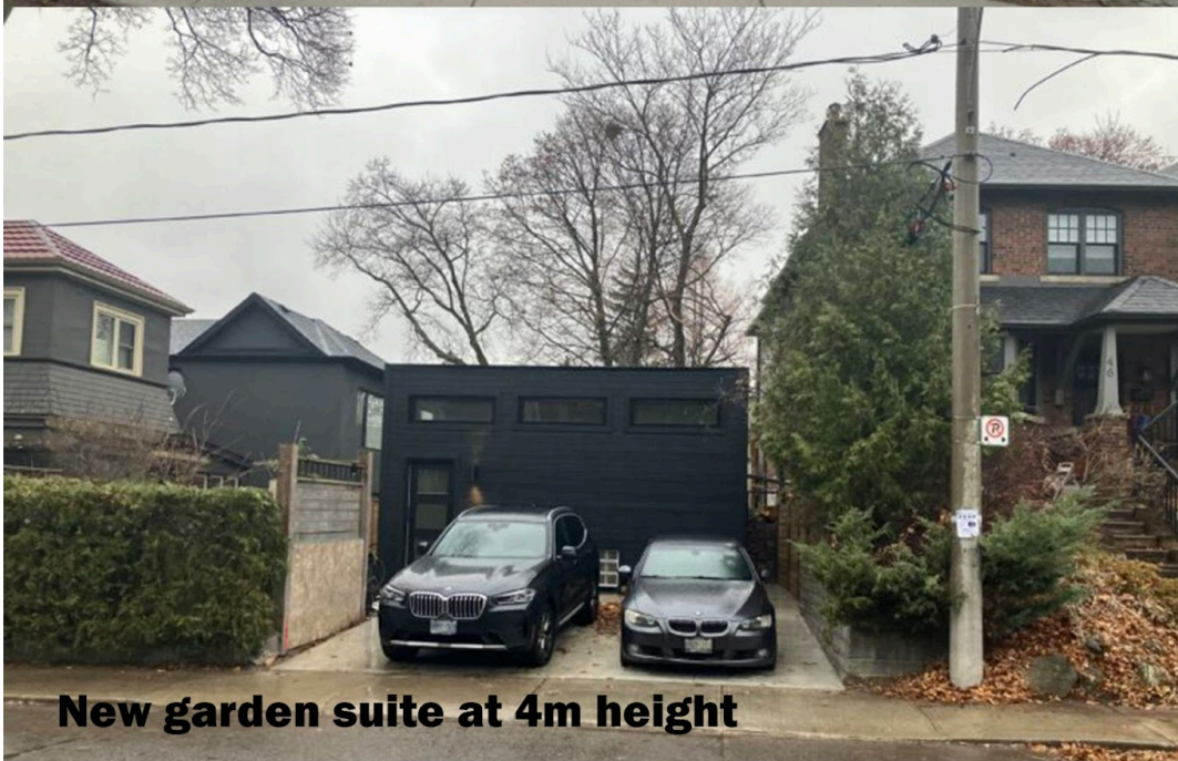
A Forest Hill garden suite converted from the existing garage footprint.
